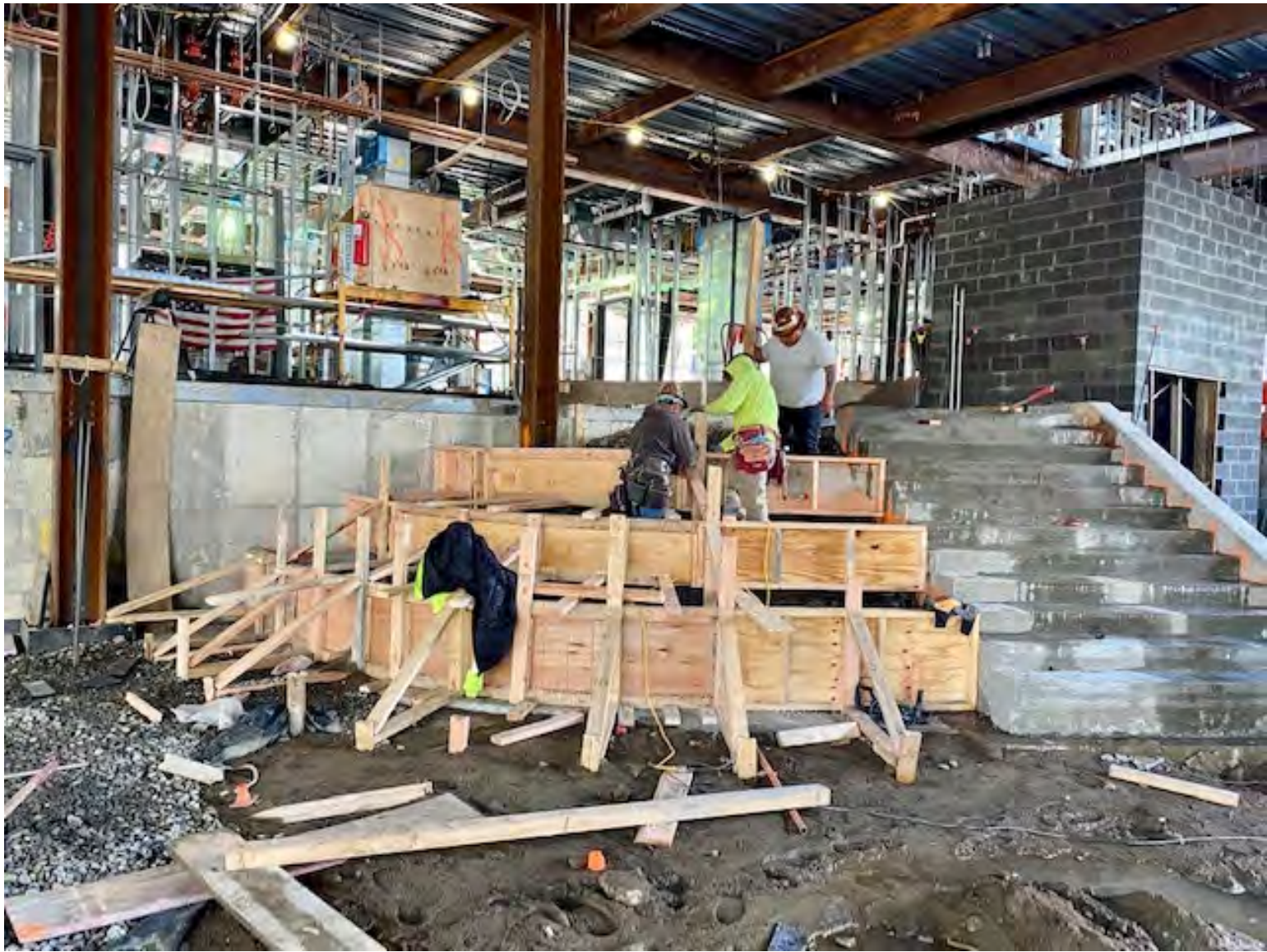
Installation of formwork for tiered seating at Cafeteria Stair E.
