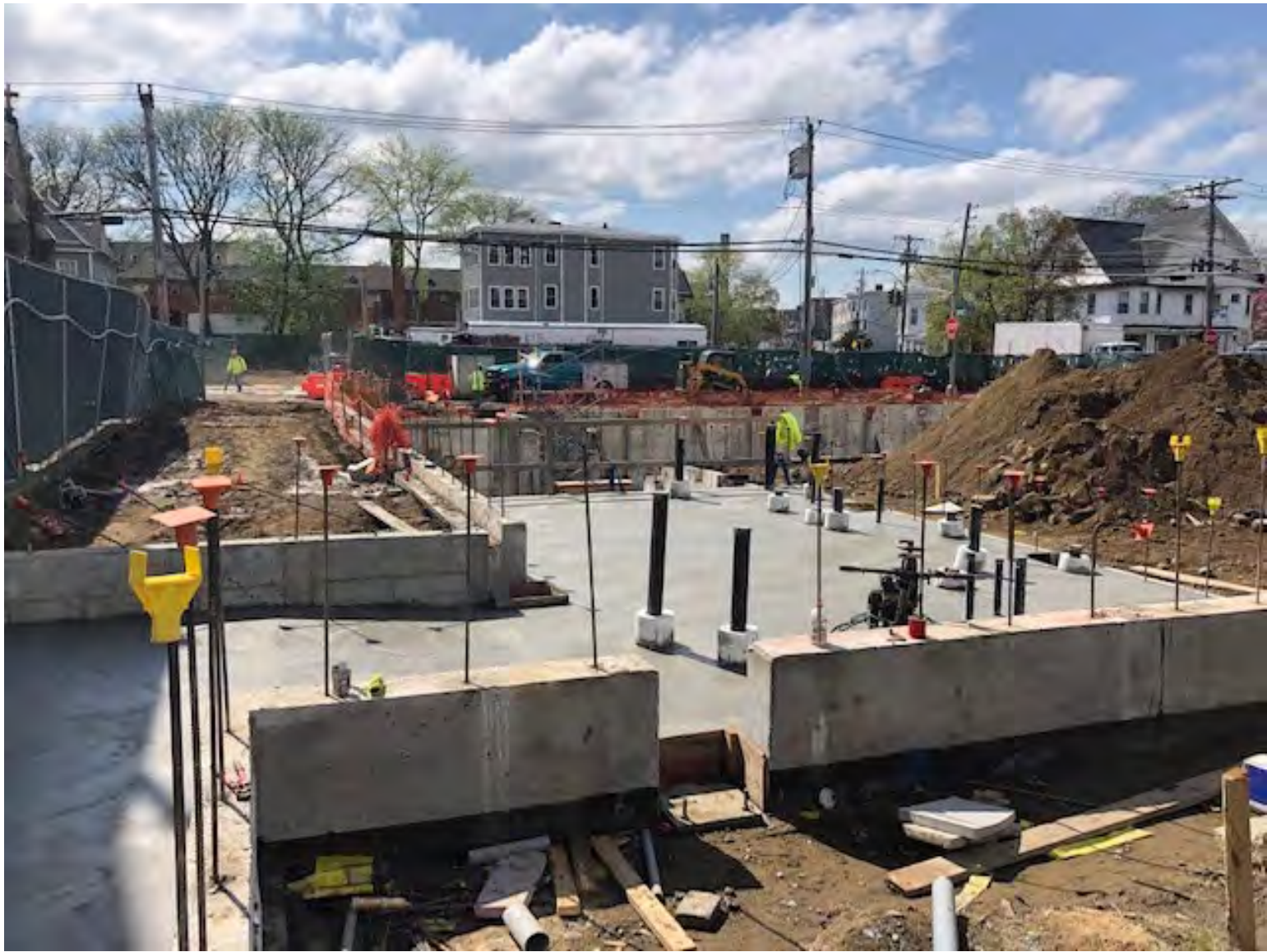
Concrete slab on grade at Community Building connector.
