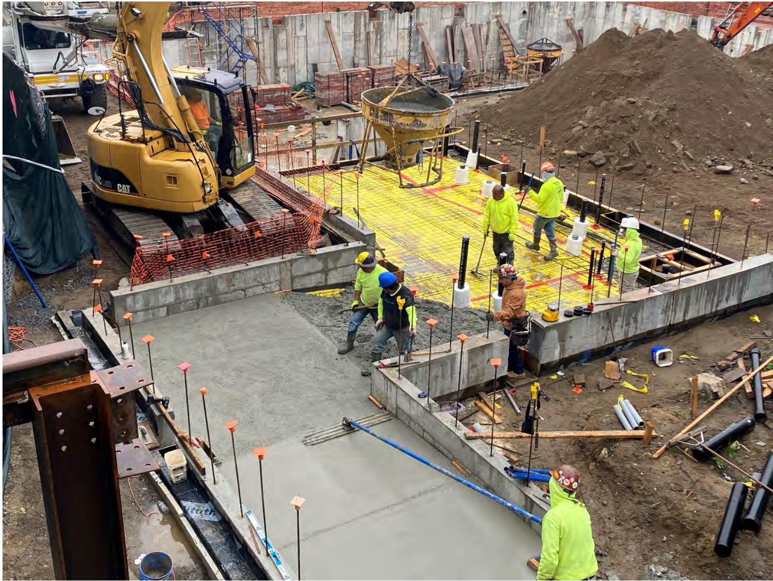
Placement of concrete slab on grade at Community Building connector.
