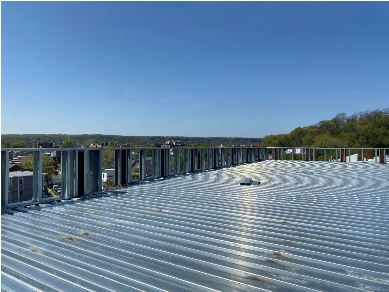
Installation of roof parapet framing at Academic Building.
