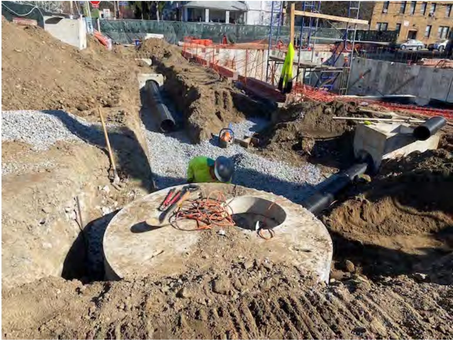
Installation of drainage structures and piping at Community Building.
