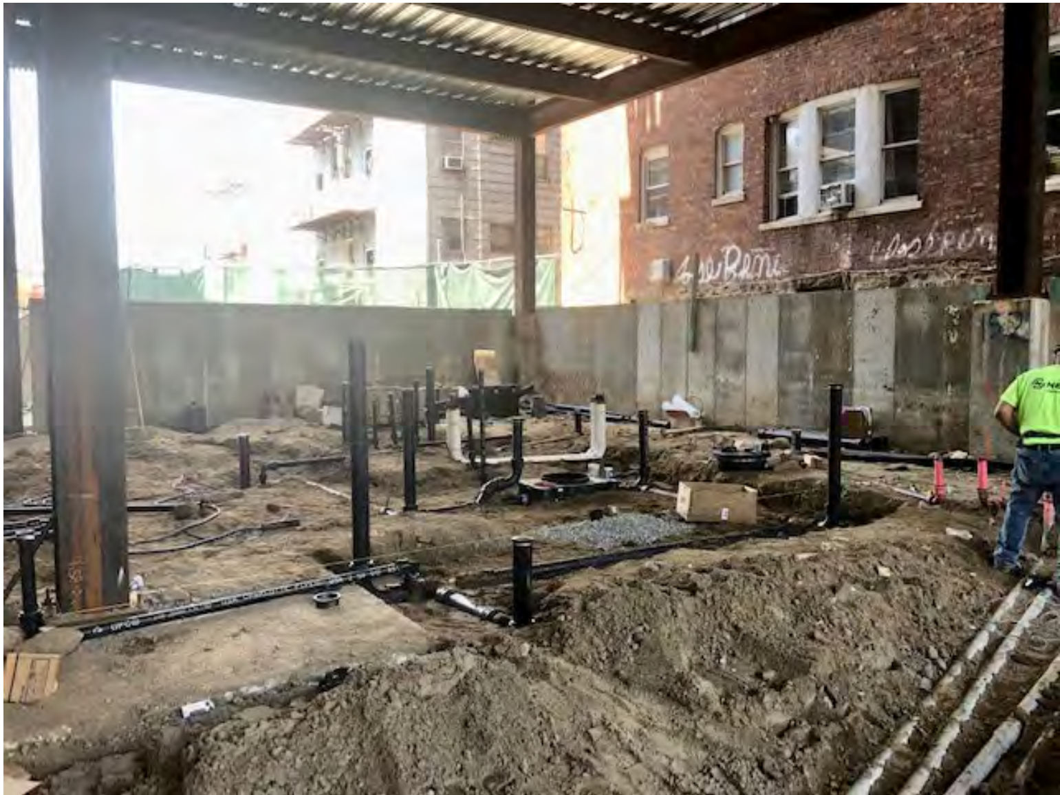
Installation of underground storm & sanitary piping at Kitchen area.
