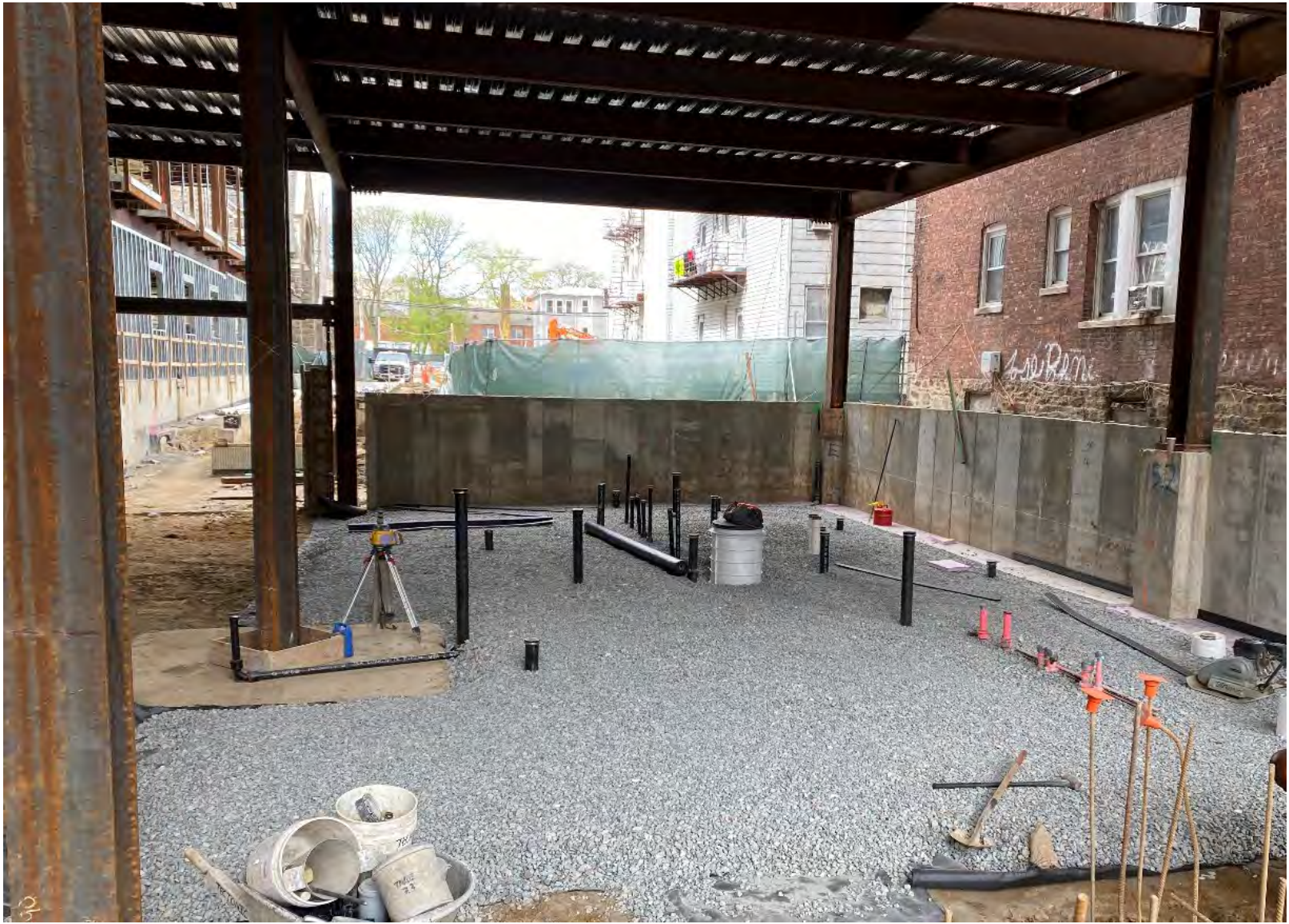
Prepare slab on grade at Kitchen area.
