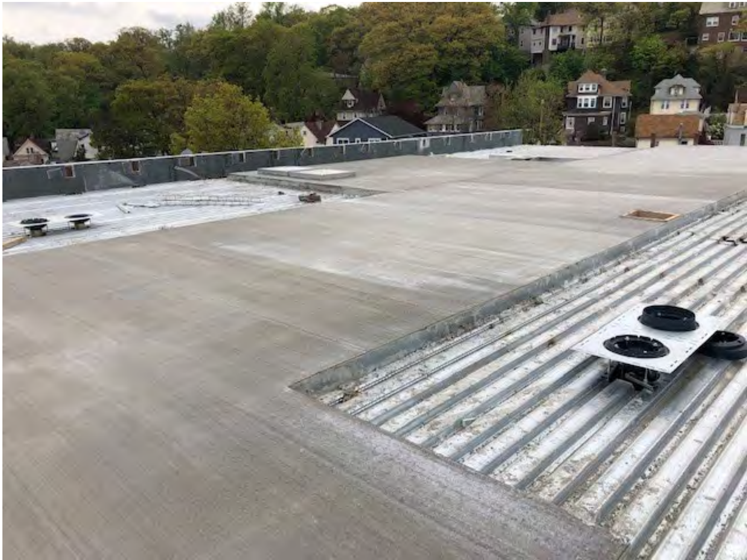
Installation of roof drains & HVAC equipment concrete pad at Academic Building.
