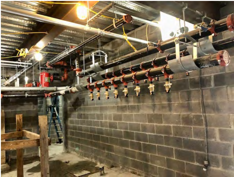
MEP equipment installation at Academic Building Basement.
