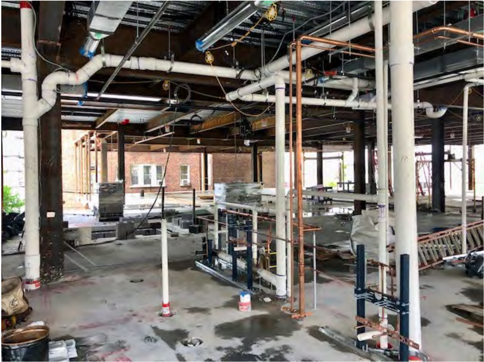
Interior MEP roughing at 2 nd floor Academic Building.
