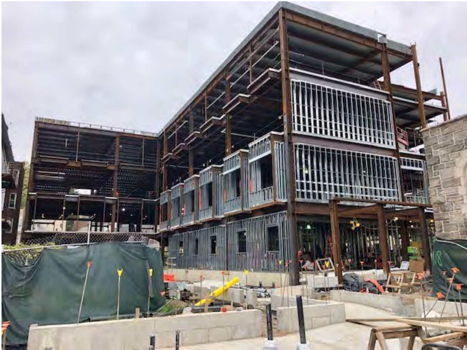
Exterior wall framing at 1 st , 2 nd and 3 rd floor Academic Building.
