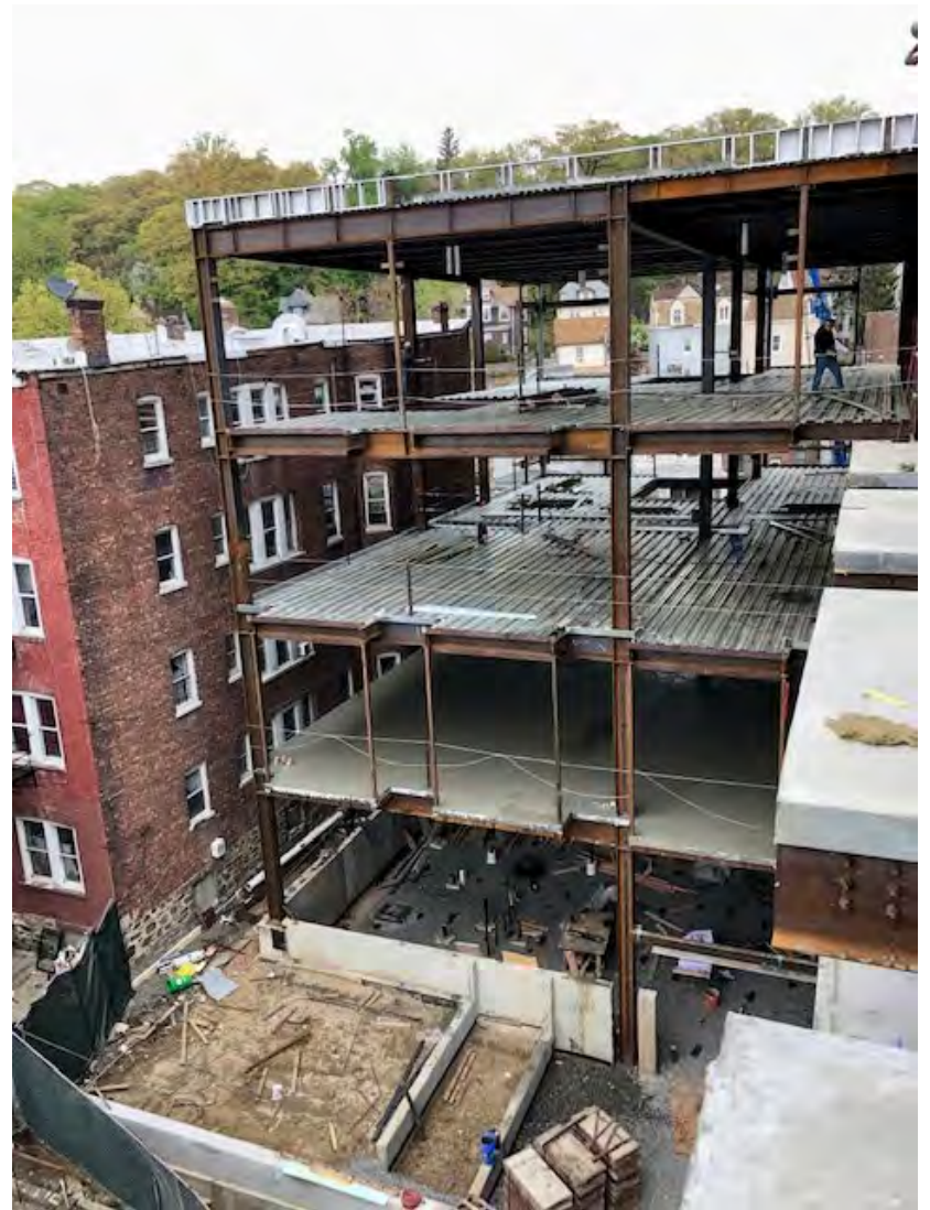
Decking and roof parapet framing at Academic Building next to 117 McLean property.
