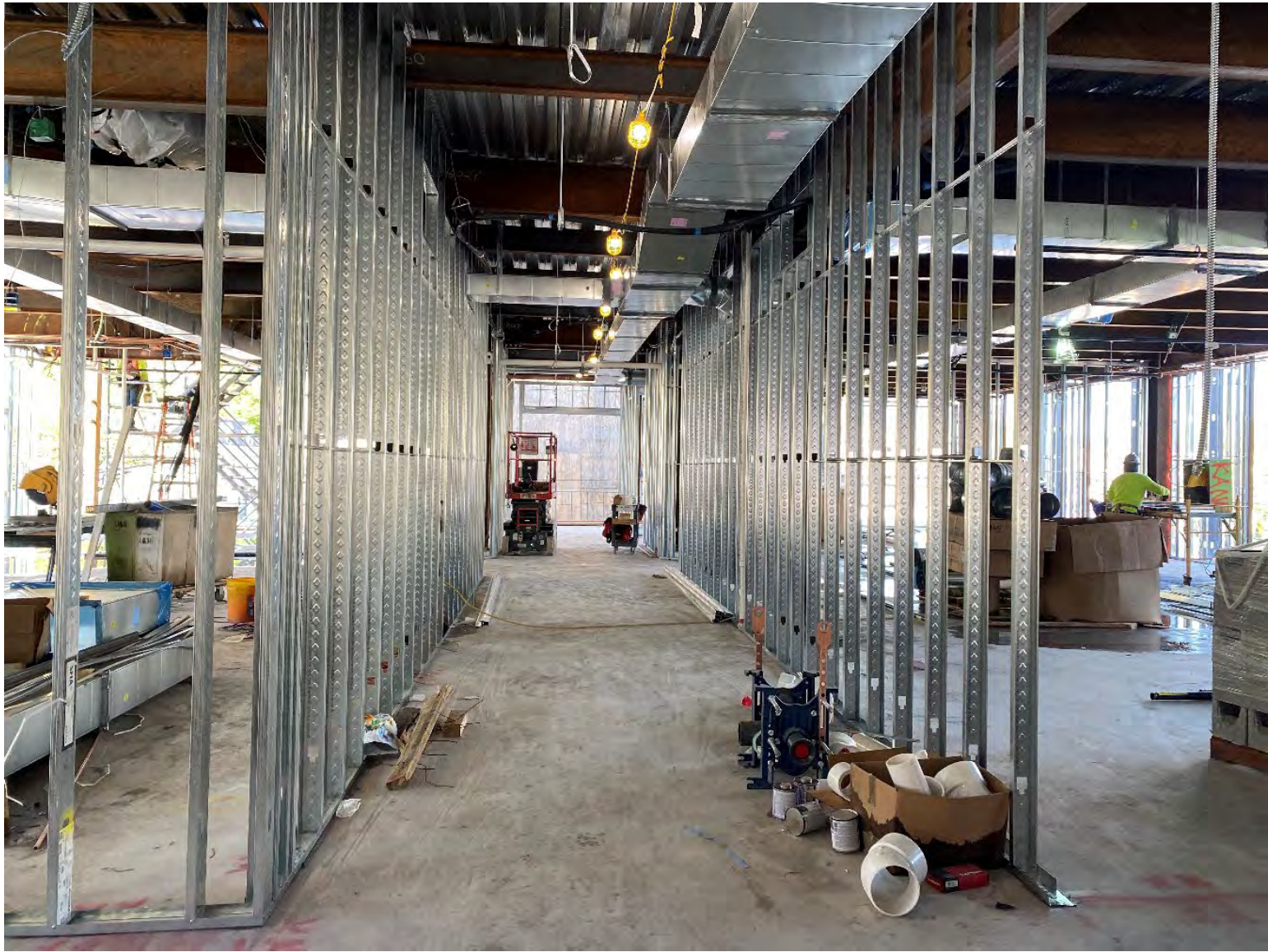
Interior wall framing and ductwork installation at 2 nd floor Academic Building.
