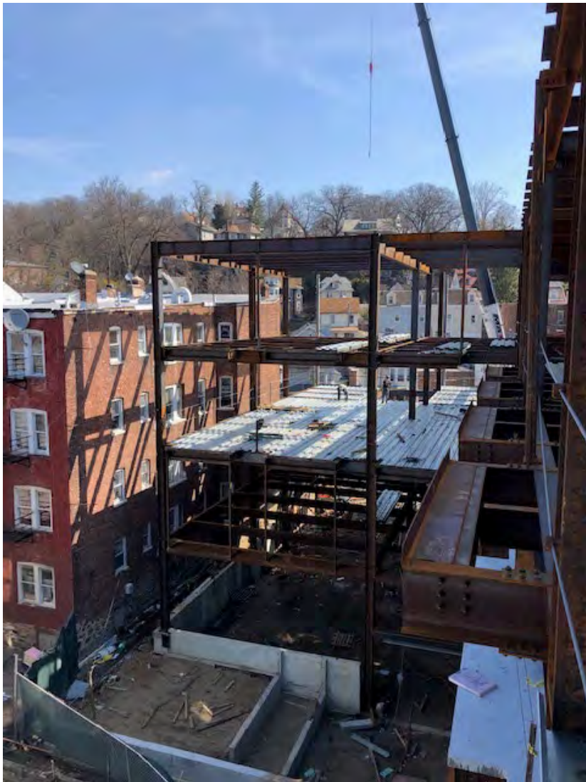
Decking and roof parapet framing at Academic Building next to 117 McLean property.
