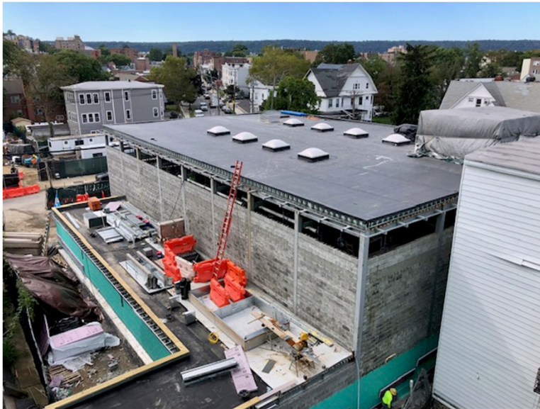
Installation of EPDM roofing system at Community Building roof.
