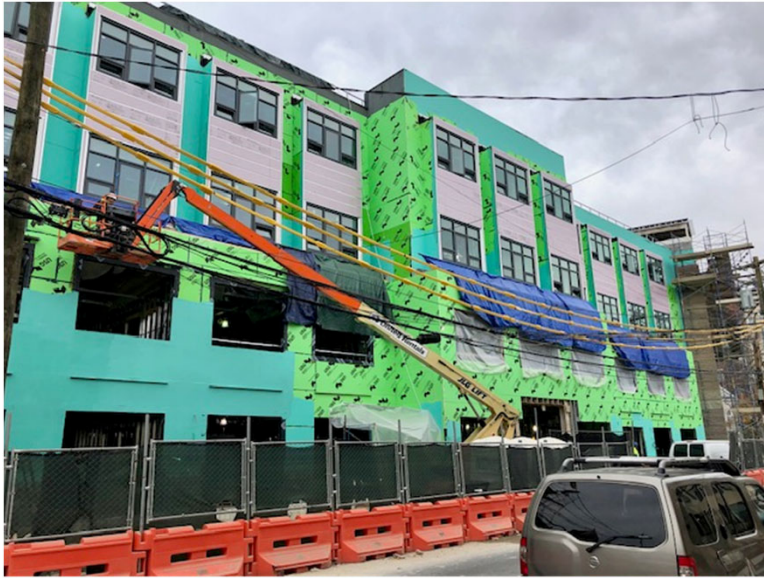
View of Academic Building looking Northeast.
