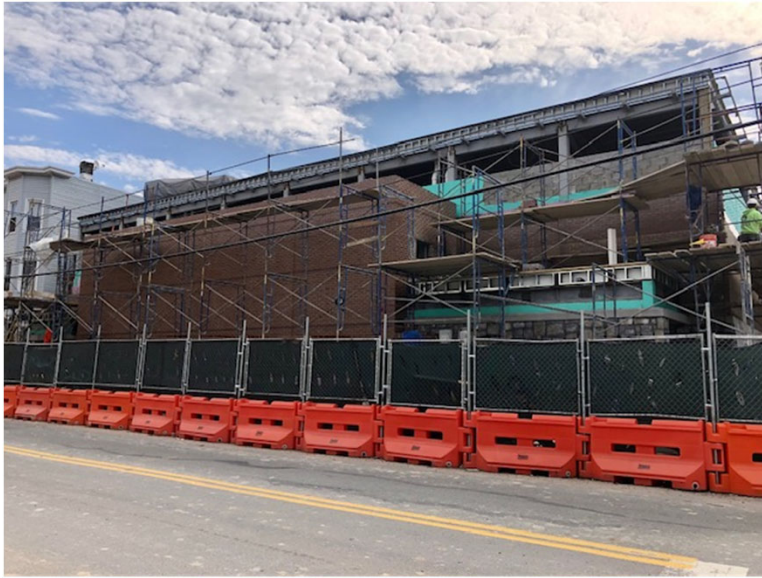
Installation of brick veneer at Community Building.
