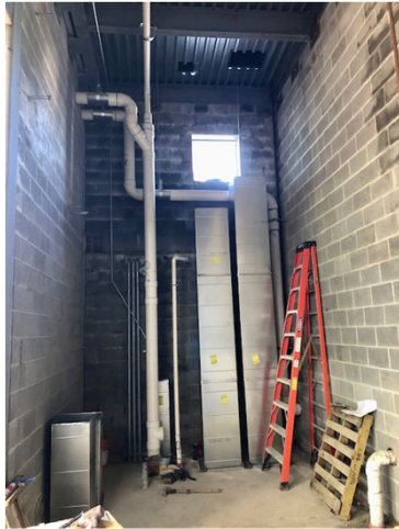
Installation of ductwork and storm piping at Community Building.
