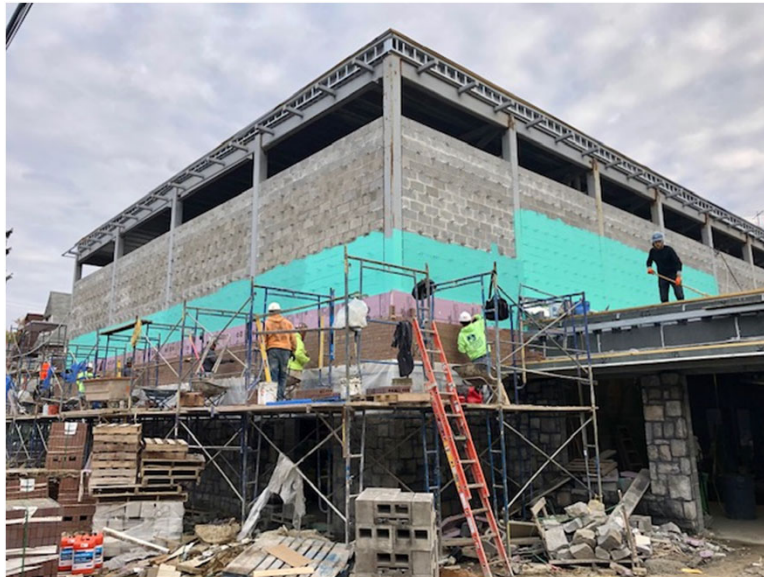
Installation of brick veneer at Community Building.
