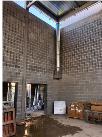
Installation of ductwork and storm piping at Community Building.
