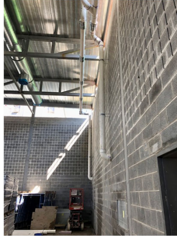
Installation of ductwork and storm piping at Community Building.
