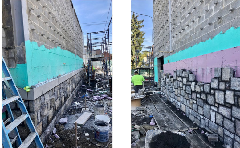
Installation of stone veneer and precast at Community Building.
