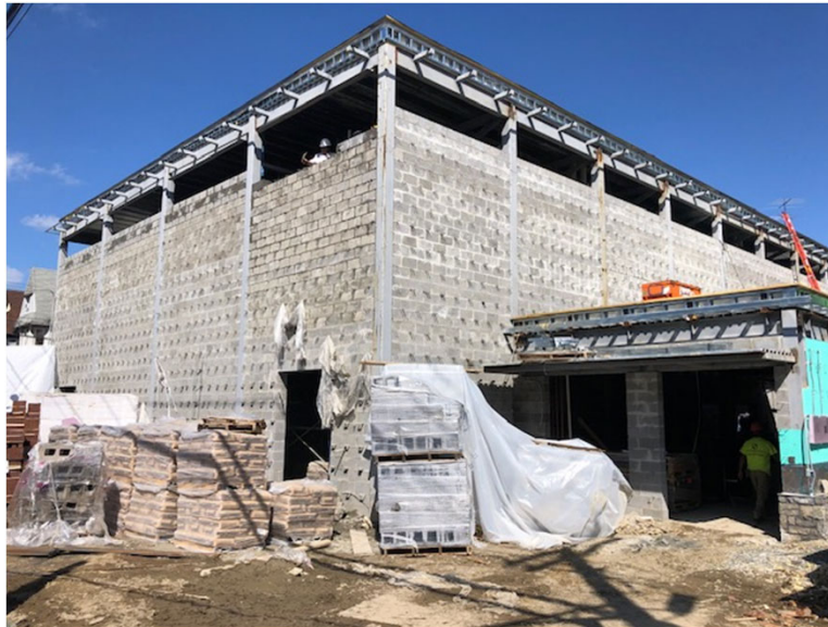
Installation of CMU at Community Building.
