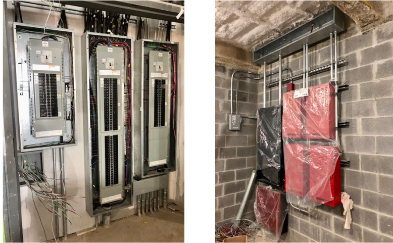
Installation of electric and fire alarm panels at Academic Building.
