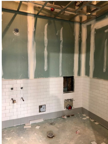
Installation of wall tile at 4 th floor toilet rooms Academic Building.
