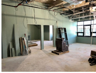
Installation of sheetrock at 4 th floor classrooms Academic Building.
