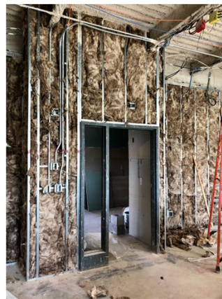
Installation of blocking and insulation at 4 th floor classrooms Academic Building.
