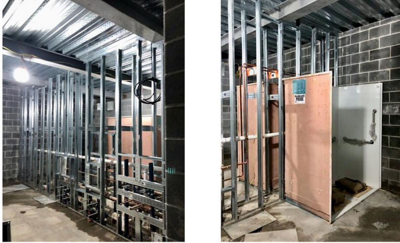
Toilet room roughing at Community Building basement.
