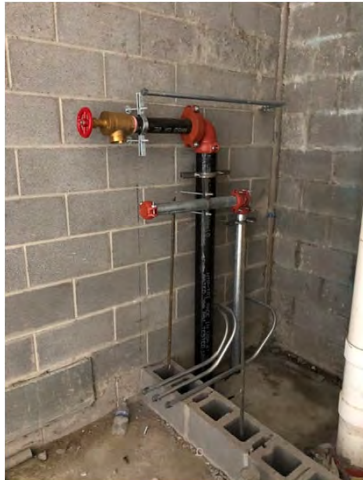
Installation of sprinkler piping and electrical feeders at Community Building.
