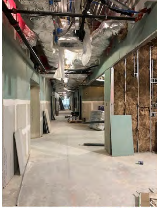
Installation of sheetrock at 2nd floor corridor and classrooms Academic Building.
