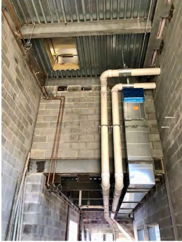
Installation of ductwork and piping at Community Building
