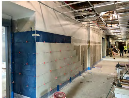
Installation of terrazzo base and wall tile at 4 th floor corridors Academic Building.
