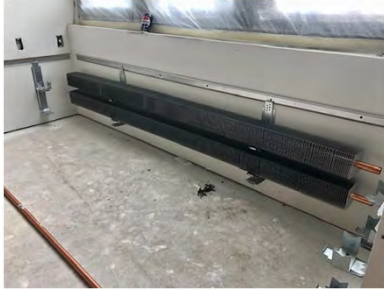
Installation of fin tube radiation & covers at 4 th floor classrooms Academic Building.
