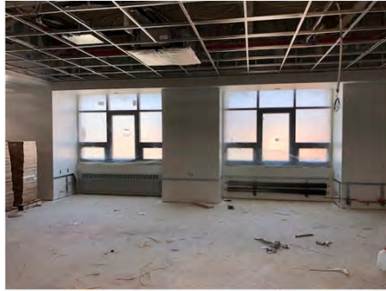
Installation of ceiling grid at 4 th floor classrooms & corridors Academic Building.
